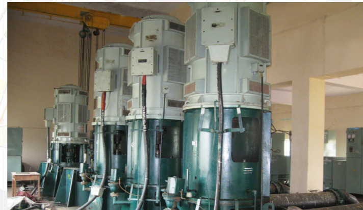
Lift Irrigation System Pumpstation
