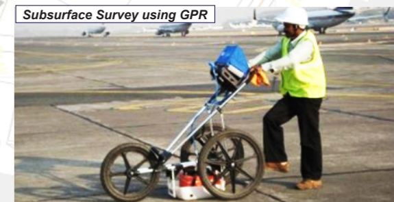
Subsurface Survey using GPR
