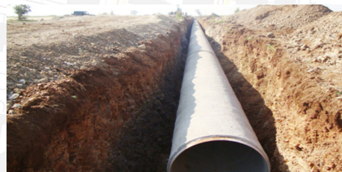
Raw Water Transport Main
